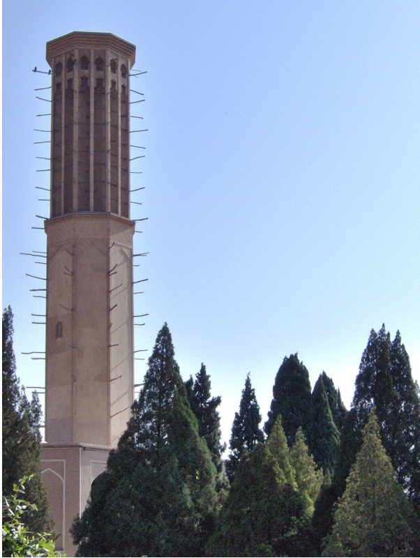
Fig. 2 The octagonal badgir of the Hashti pavilion at Bagh-e Dolat Abad
