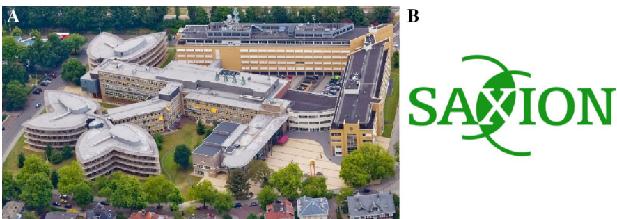
Fig. 6 Both the Saxion University in Enchede designed by Paul Dirks (a) and the Logo of the University (b), are based on the Vesica Piscis design
