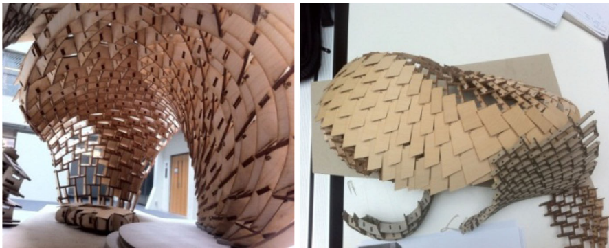
Fig. 5 Two views of the reciprocal structure realized by the students at the University of Melbourne in 2012. The nodes and construction have adopted the same principles used for the Serpentine Gallery 2005
