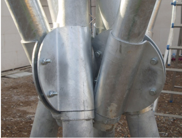
Fig. 19 With the correct position of bars indicated by means of a ring around the pipes
