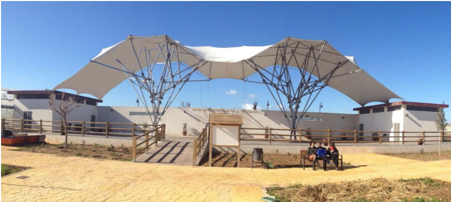
Fig. 25 Lateral view of the finished roof
