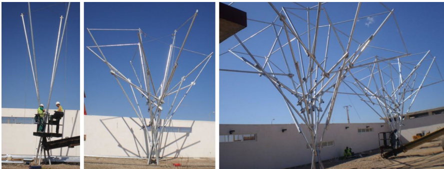
Fig. 20 The installation of tree structures
