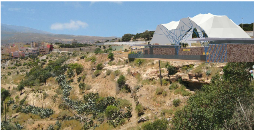
Fig. 10 Initial design for a Centre for Nature Interpretation in Melilla, North Africa
