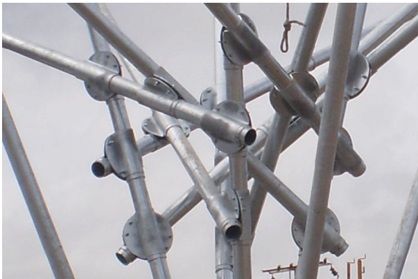
Fig. 18 Group of joints solved with disc plates to connect bars
