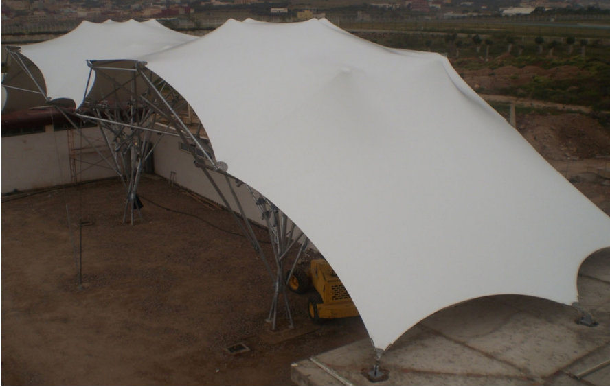
Fig. 24 The finished roof in January 2011
