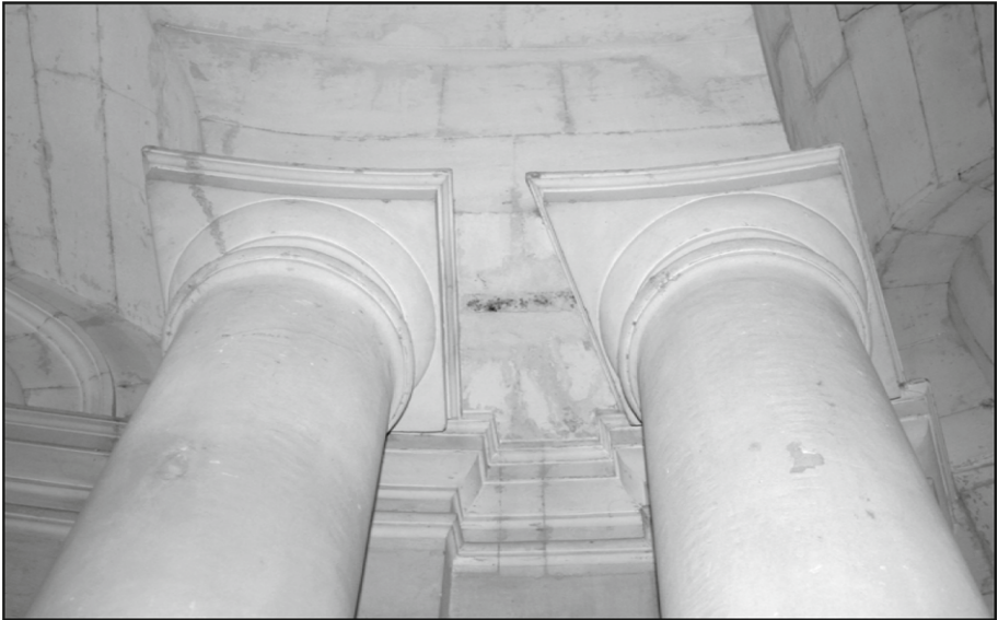
Fig. 10. Close-up of the capitals showing their actual distorted form
