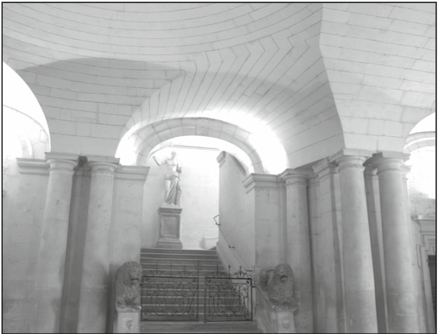
Fig. 15. The striped surface appears to be divided into two different parts from the keystone. Looking along the line passing through this voussoir, which separates the two portions of the conoid, it appears that the point of convergence of the straight lines falls exactly on the median axis of the wall at the bottom of the stairs, where is the statue of Venus is located, while the two conoids could have two different vertices, on the axis itself
