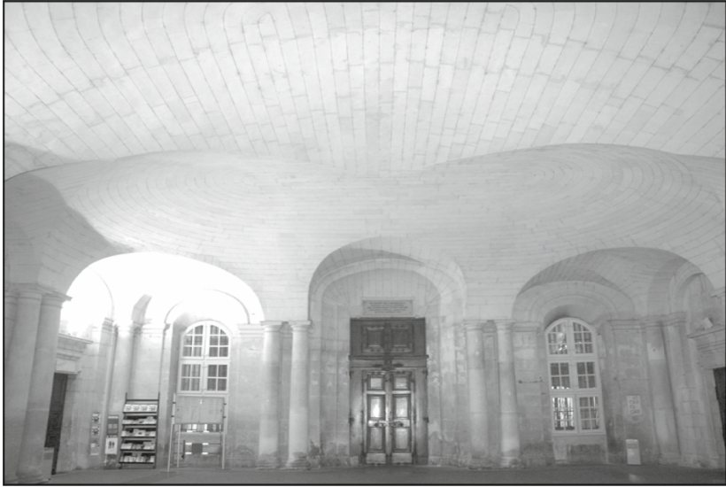
Fig. 13. Seen from the main entrance, the vault seems to have very shallow rises to “fall” heavily on those who pass through the south entrance. The optical effect is due to the continuous horizontal lines on the large vault, which create a strong sense of “crushing”
