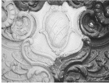
Fig. 7. Stucco from a chimney (appr. 1890) cleaned at 1064 nm ( left part )
