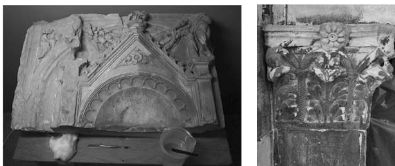
Fig. 2. On the left: Fragment of the Fonte Gaia (Siena), with a partial laser cleaning; on the right: Typical black encrustations on the façade of S. Pietro in Vincolis (Pisa)
