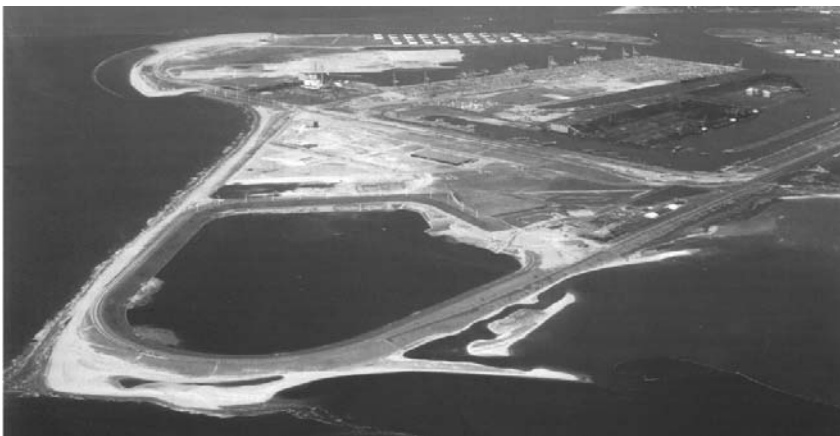
Fig. 2. The Slufter – a confined disposal site for contaminated dredged material
