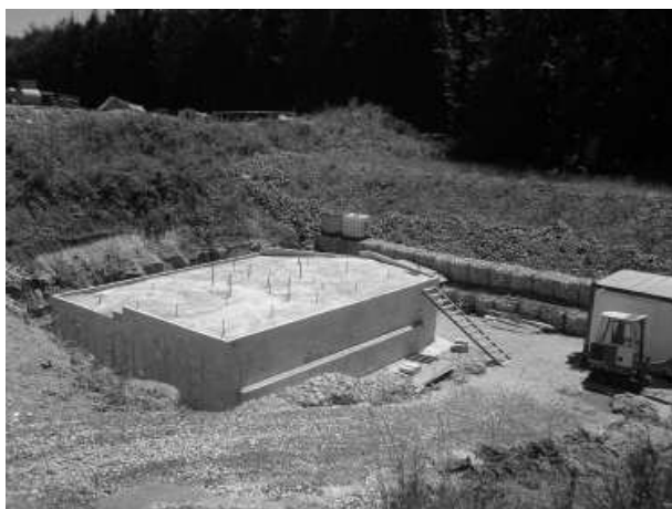
Fig. 5.10. Completely encapsulated field block; direction of view: south-east.
