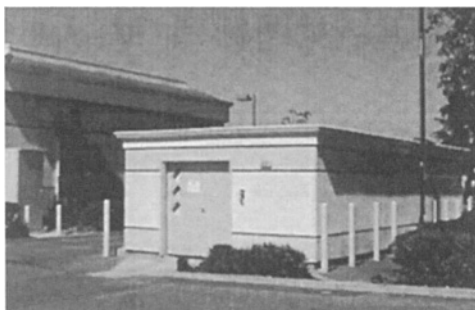
Figure 8. Photograph of the HiPOx installation at the Northern California gas station
