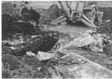
Figure 5. Uncovering the UST during the 1999 Pre -Design Investigation, note the oily (dark) quality of the subsurface soil
