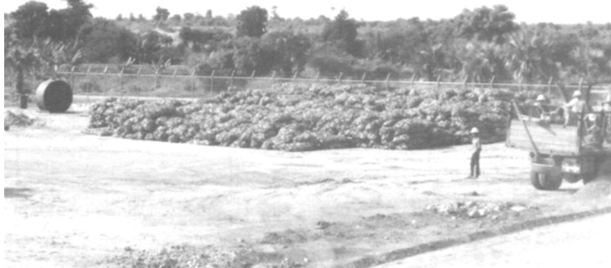
Figure 1 — In-settler medium in 1-m 3 bags for installation in a large copper settler (total volume 120 m 3 ).
