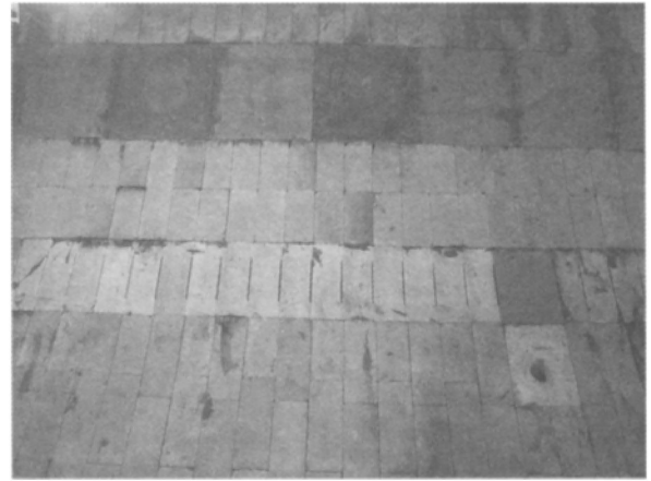
Figure 10 — Slots and fines return brick.
