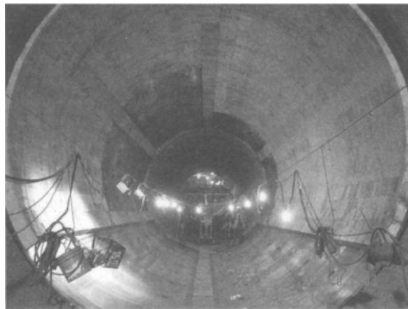
Figure 9 — Installing refractory.
