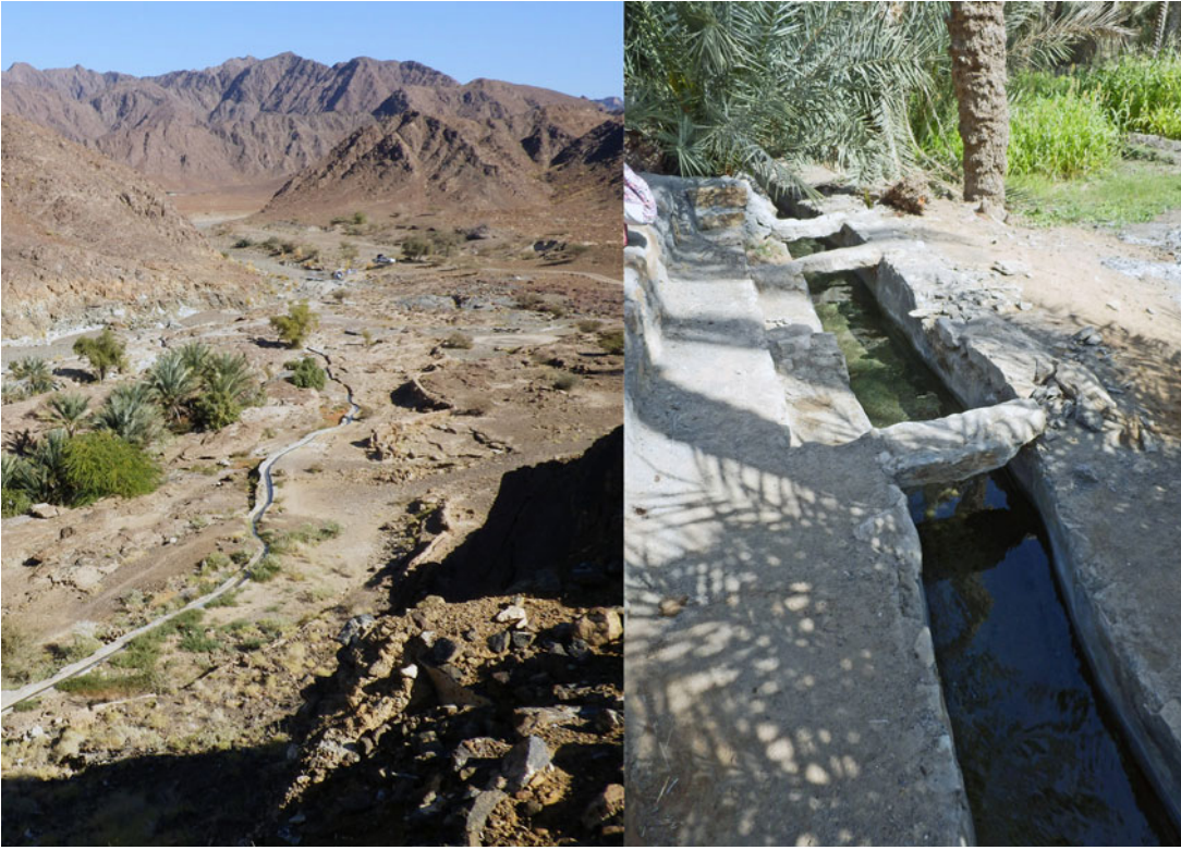
FIGURE 1. Left : A falaj channel in a wadi valley, Al Banah, Oman; and right : a falaj irrigation channel in central Bat, Oman. While these examples are from Oman, falaj are common in much of the Middle East. (Photos by Alasdair Brooks, 2015.)
