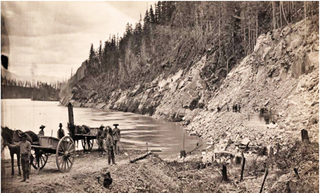
FIGURE 2. Chinese railroad construction workers building the Northern Pacific Railroad grade along the Clark Fork River, ca. 1882. (Oregon Historical Society Collection, Image 002822.)
