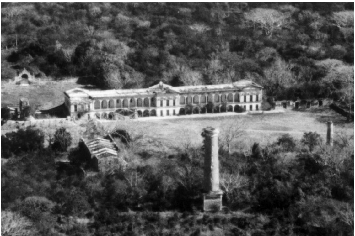
FIGURE 3. Tabi's principal house, with church and sugar mill chimney in the foreground. (Courtesy of the Cultural Foundation of Yucatán, Mérida, Mexico; photo by E. Logan Wagner, 1992.)
