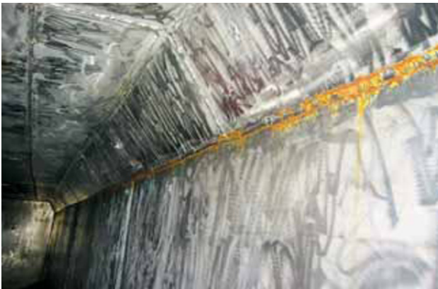
Figure 1 – Image from the inside of a fishing boat showing coarse ground surface attacked by corrosion
