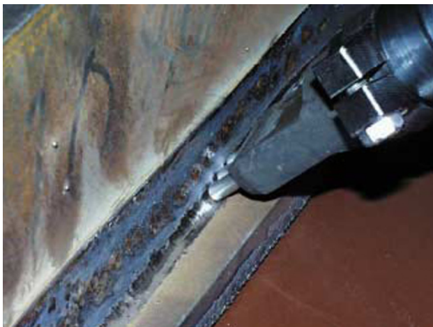
Fig.2. The performance of ultrasonic impact treatment.
