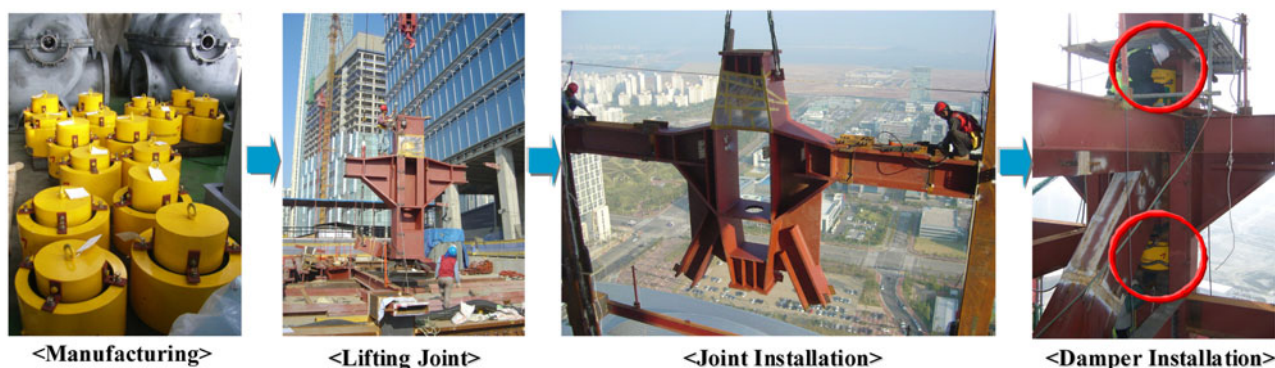
Figure 11. Installation of manufactured outrigger dampers.
