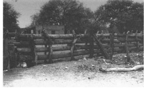
Fig. 5. Corral of Sabal uresana logs, Rancho La Noria Aguilareña, Mpio. Ures, comprised of approximately 200 logs cut ca. 10 years ago from standing dead palms on the ranch.
