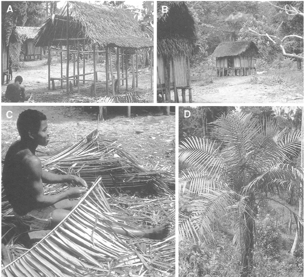
Fig. 1. Dypsis fibrosa . A. Construction of a roof with D. fibrosa leaves. B. Completed house. C. Preparation of thatching panels from leaves. D. Habit (All photos by J. Dransfield, 1986).
