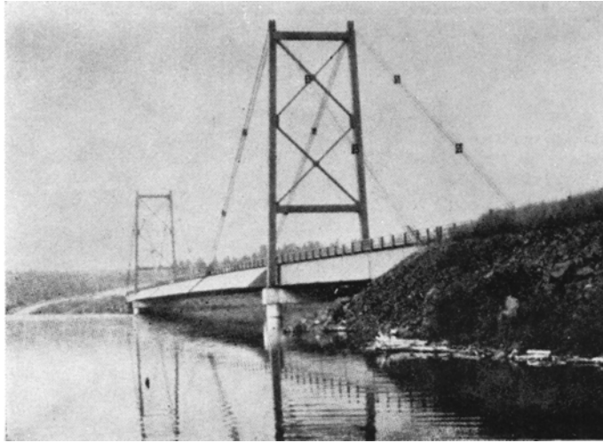
Figure 9. The modified Long's Creek Bridge
