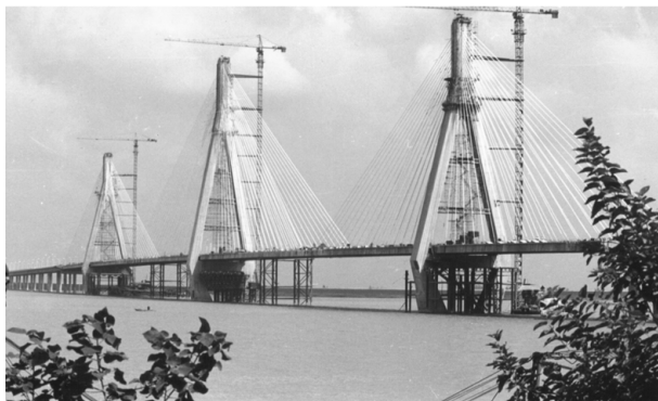
Fig. 18. Cable-Stayed Dongting Lake Bridge
