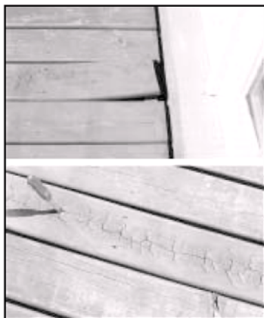
Figure 8—Warping (top) and excessive surface degradation (bottom) resulting from juvenile wood.
