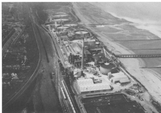
Fig. 12—Aerial view of sea water magnesia plant at Hartlepool. (Courtesy of Steetley Company).
