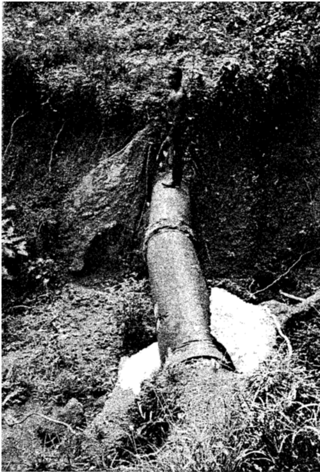
Fig. 2 : A. Northern section of the damaged pipeline at Bromley Hill.
