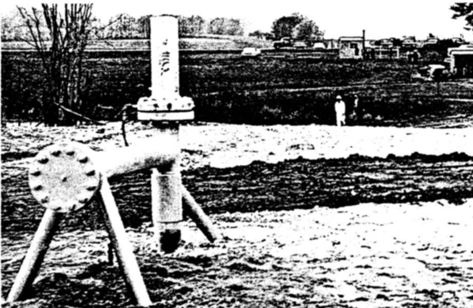
Figure 1. Arrangement for discharge of vertical jets in 1965.
