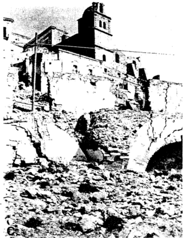
Figure 1. Landslide damage of grades 5, 6, and 7 in Italy: A. Hospital in reinforced concrete, Ancona (grade 5). B. Houses in rubble masonry, Tricarico, Matera (grade 6). C. Total destruction of the urban environment, Craco, Matera (grade 7).
