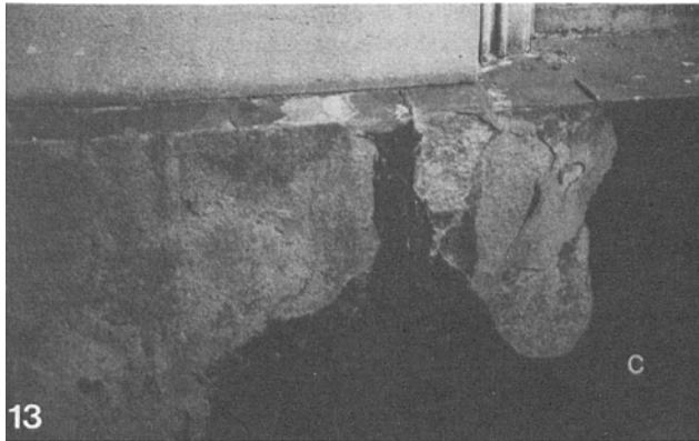
Figure 13. Spalling of thin slabs of granite in several layers. Base of Tweed Courthouse, Lower Manhattan, New York.
