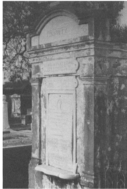
Figure 12. Slab of fine-grained Italian White marble, weathered and warped after exposure of about 100 y to 2000 mm precipitation and high relative humidity of New Orleans, Louisiana.
