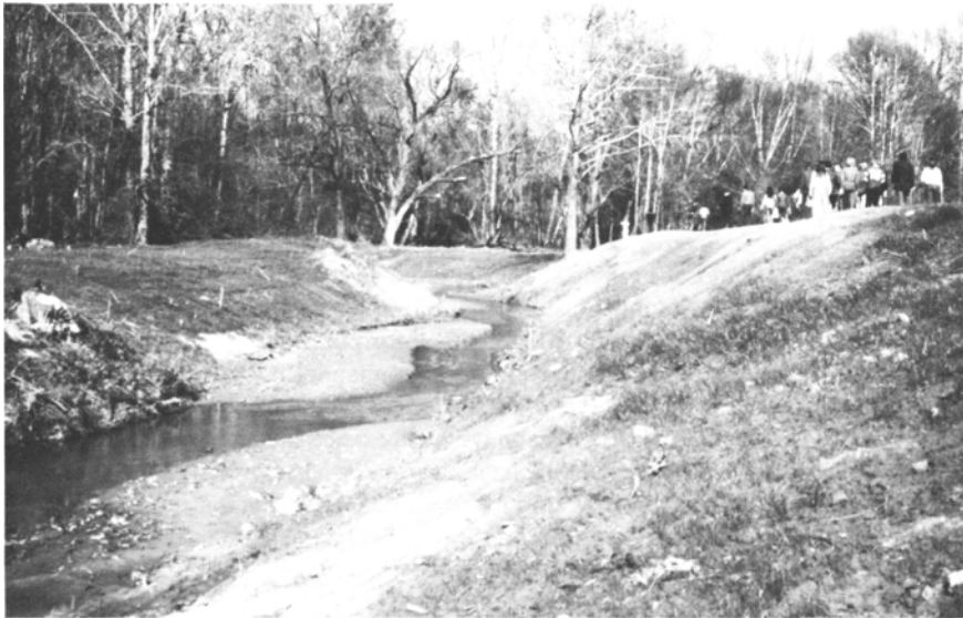
Figure 6. Series of bars that developed in Gum Branch as designed. Compare the actual morphology with the idealized morphology of Fig. 4.
