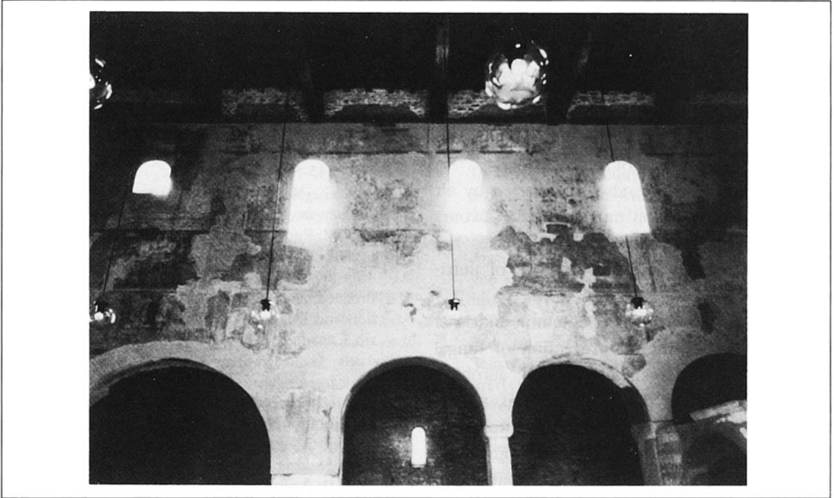
Figure 1. Mural paintings covered by black patina due to Cladosporium growth - Basilica of S. Vincenzo, Cantù (Como - Italy).
