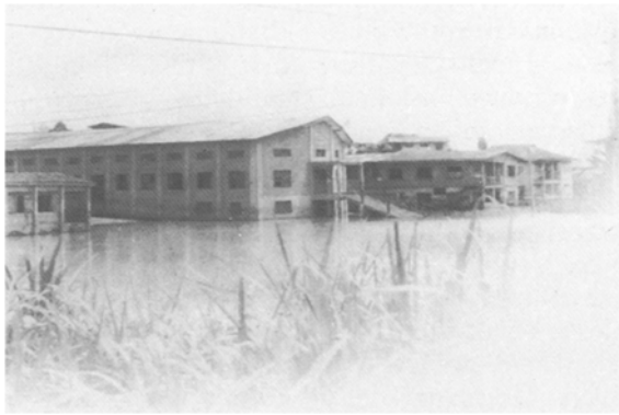
Fig.2 Street flooding in the study area; Ondo, Nigeria.
