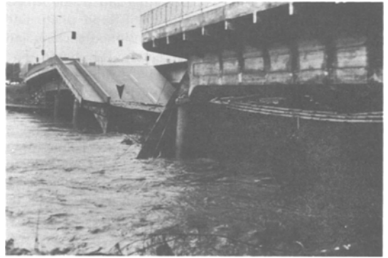
Figure 11. Failure of one downstream span of the Soquel Avenue bridge. Note high water mark. Scour led to settling of an older pier supporting the down stream span.
