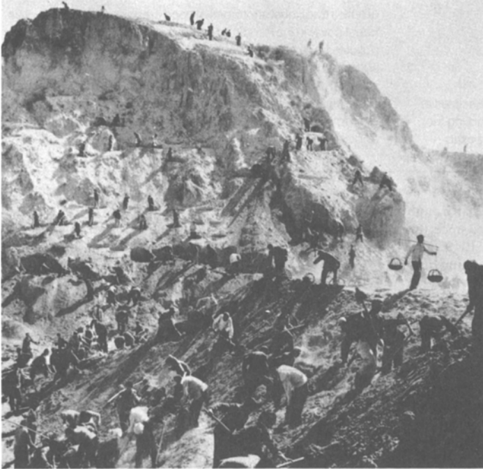
Figure 1. Peasants in Hequ county in northern Shanxi province building new terraced fields in loess deposits with traditional Chinese tools—pickaxes, shovels, shoulder poles, and baskets.
