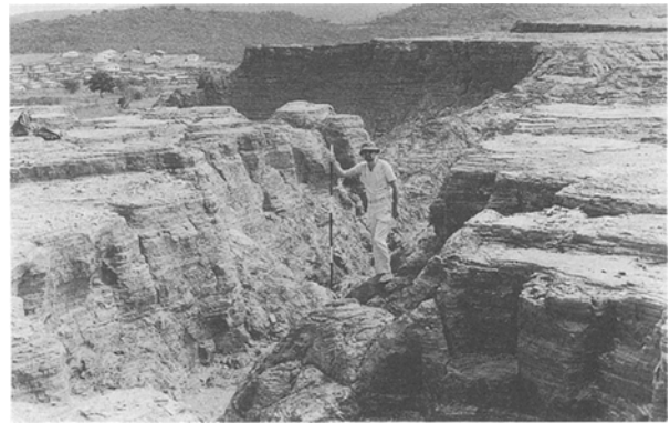
Figure 12. Deep gully that formed at the time of failure in wet tailings. The slumping of the originally wet tailings on the margins of the gully can be seen.
