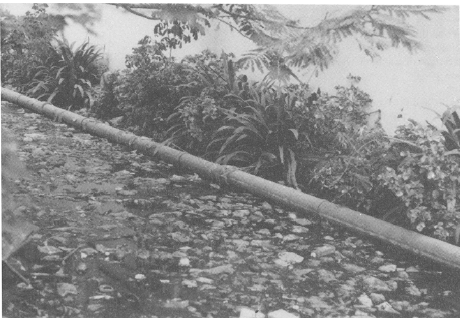
Fig.5 The necessity of maintaining a positive chlorine residual in water supply pipe lines is emphasised, for here in Bangkok, Thailand, the pipe passes through a sewage contaminated drainage canal.
