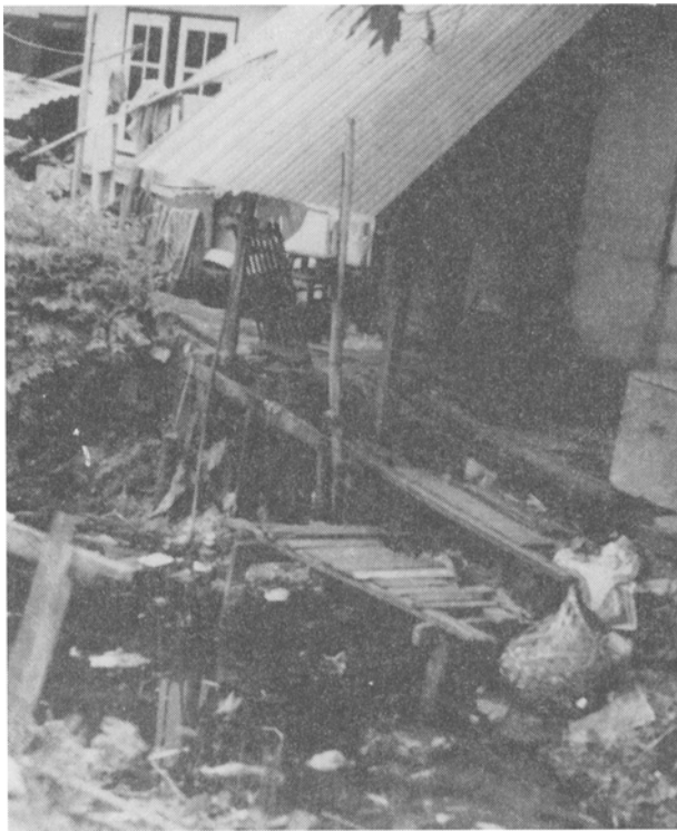
Fig.1 Poor community housing in the heart of Bangkok, Thailand. The area lacks proper drainage, sanitation or solid waste management.
