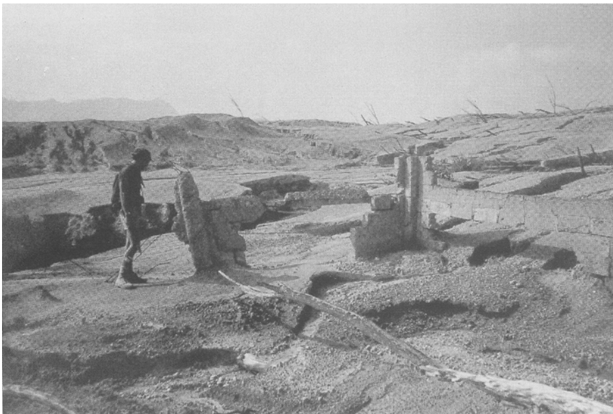
Fig. 1. Typical destruction by surges of cinder block and concrete structure in the village of San Isidoro Tanchichal, 4 km southwest of the crater. Deposit is 1 m thick. Note field of sand waves in background
