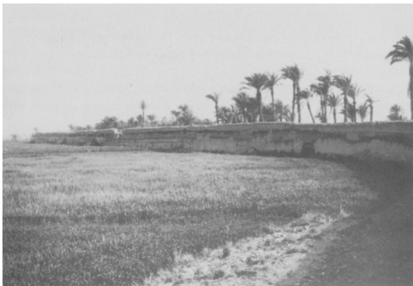
Fig. 9. Dam at Lahun separating the Fayum Depression from the Nile Valley
