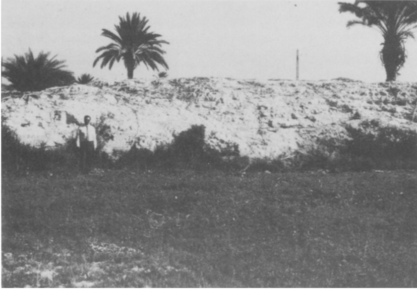
Fig. 11. Masonry Dam (downstream face) near Itsa.
