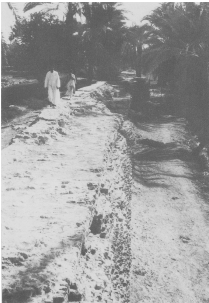
Fig. 10. Masonry Dam near Itsa (Fig. 8).
