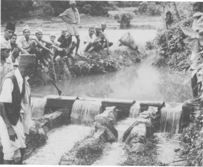
Fig. 4. A saacho installed to distribute the flow from a main canal into four secondary canals according to the water allocation of each.
