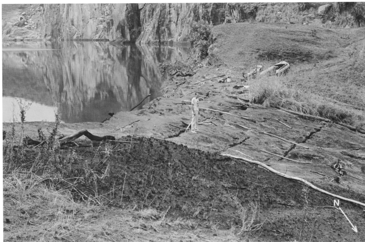
Fig. 4. Upper surface of dam, showing well-developed joints. View southwestward
