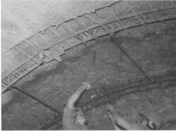
Fig. 1. Tunnel excavation with lattice girders
