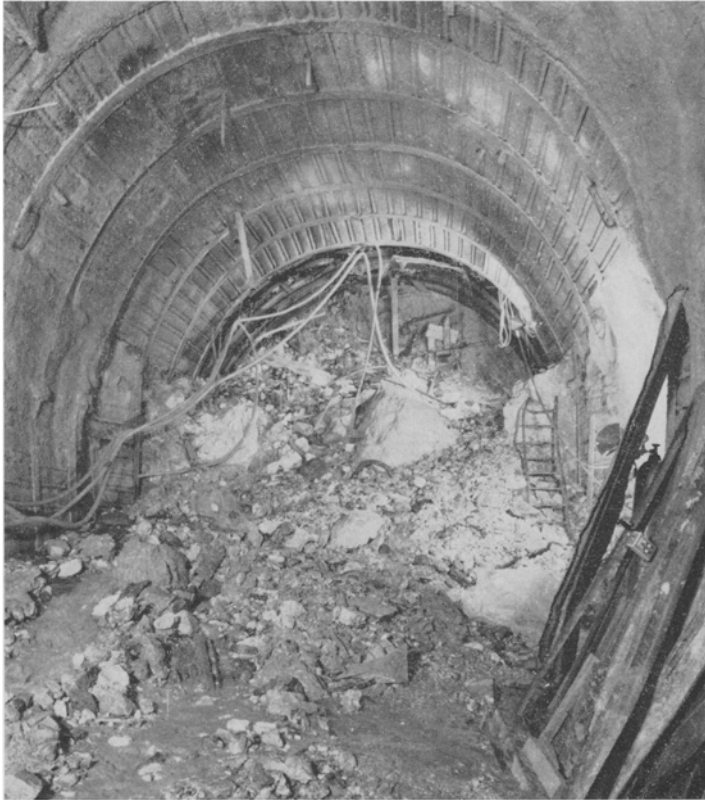
Fig. 6. Flow of crushed material and water at TM 3385
