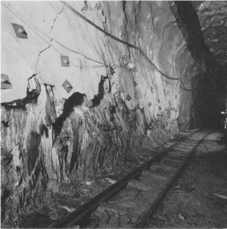
Fig. 7. Buckling of vertical layered rock
