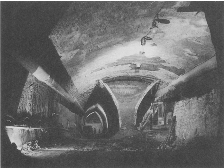
Fig. 20. Side drift method for large tunnels ( A=75-150\text{ m}^2 ) in the Tertiary
