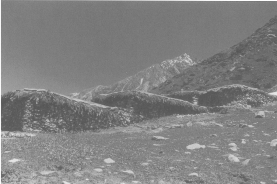
Fig. 6. Indigenous dwellings in an avalanche runout at 3300 metres elevation in upper Saiful Maiuk Valley. The construction is of stone and timber. Building the uphill wall flush with the slope reduces damage from avalanches.
