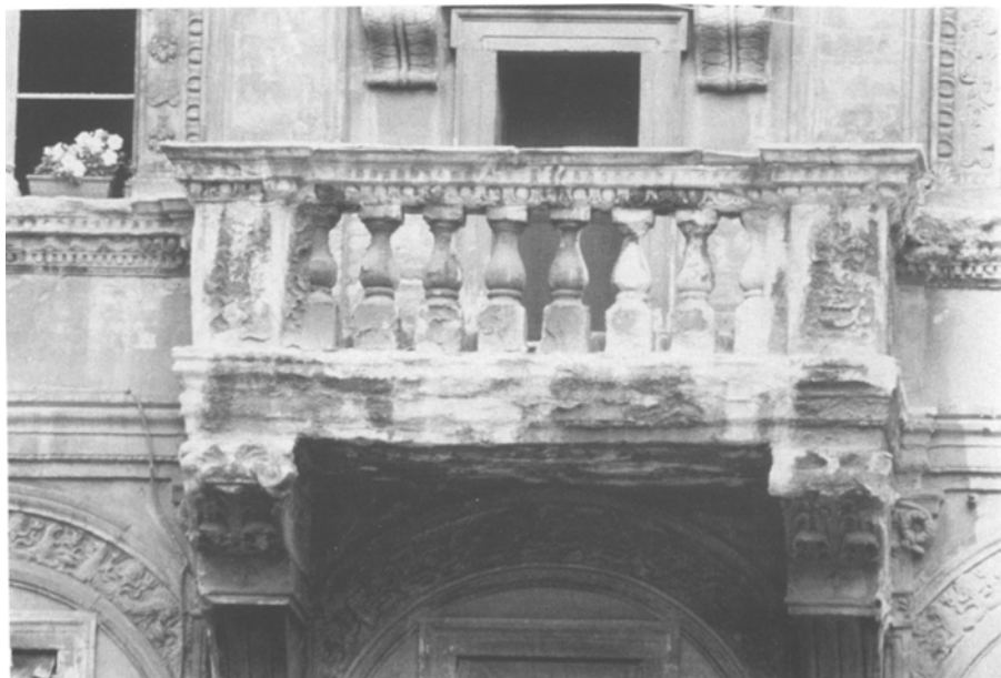
Fig. 2. Black patterns as can be observed on the surface of porous natural stones, such as calcarenites and sandstones.
