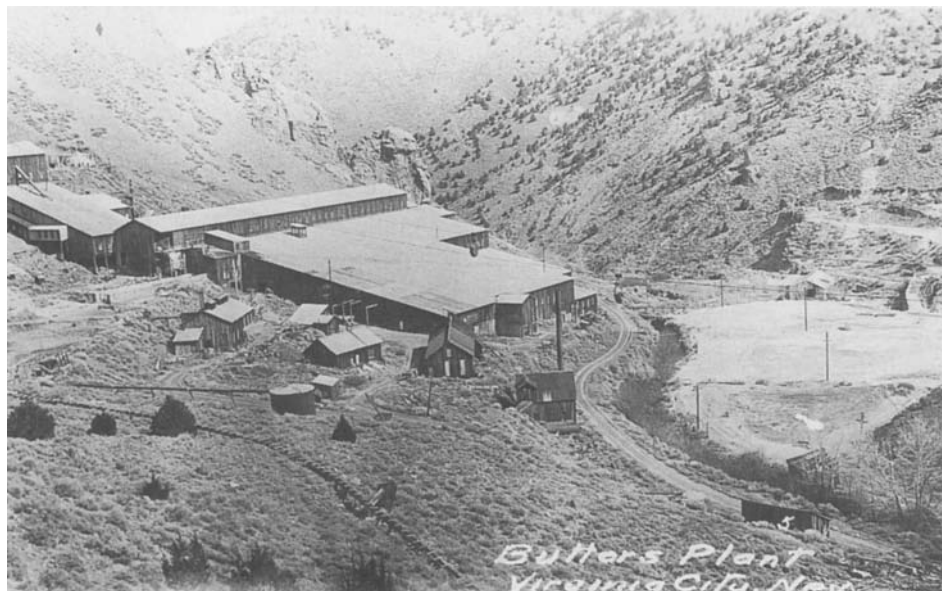
Fig. 2. A stamp mill in Sixmile Canyon. Note the light-colored tailings materials near the drainage on the right side of the photograph.
