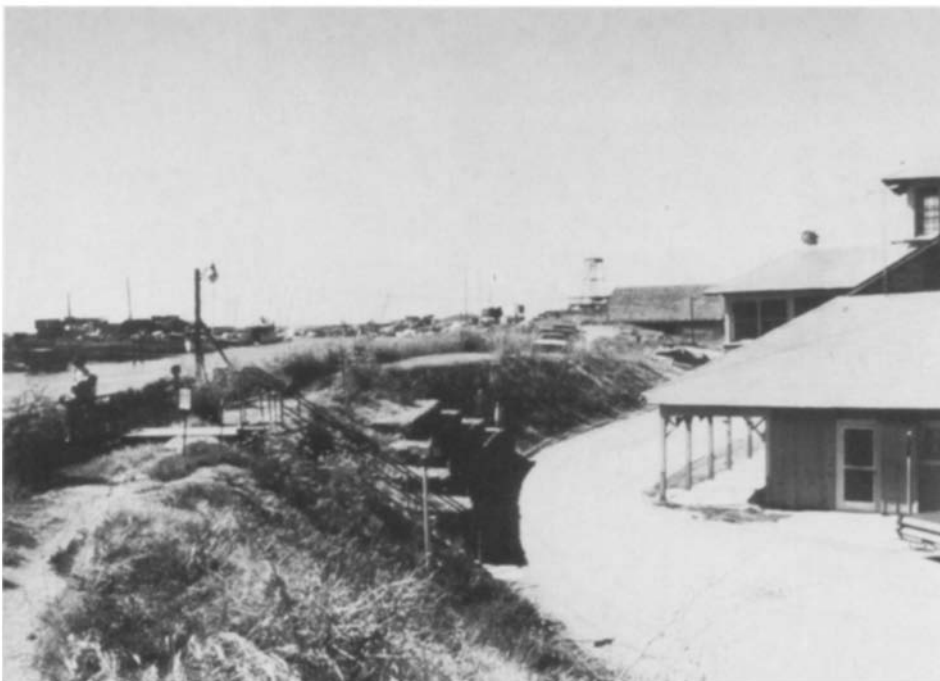
Fig 9 Alviso Yacht Club, south end of San Francisco Bay, San Jose, United States (August 1980). Area has subsided approximately 2m and is protected from inundation by levee shown in photograph. Note water level behind levee
