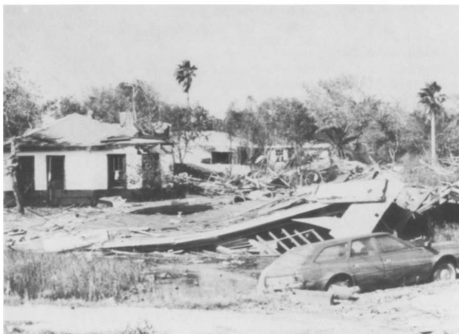
Fig 4 Houses damaged or destroyed by storm surge caused by Hurricane Alicia, Houston, Texas (August 1983)
