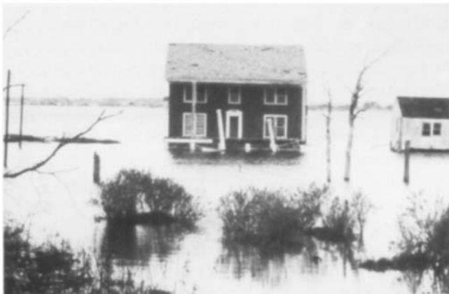
Fig 2 Abandoned house in Galveston Bay, Houston, United States (1976). Subsidence has caused bay to encroach over foundation (courtesy of C. W. Kreitler)
