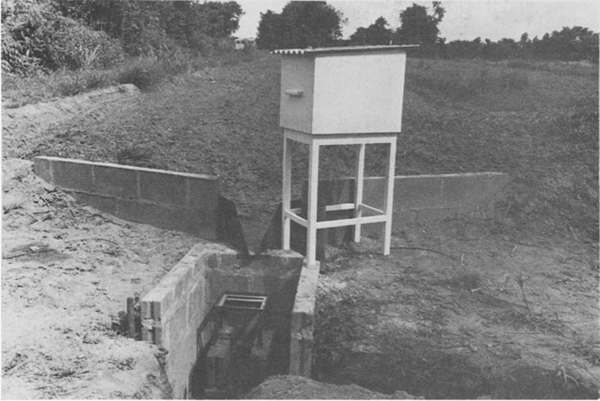
Fig. 2. A close up of the collection system looking upstream.
