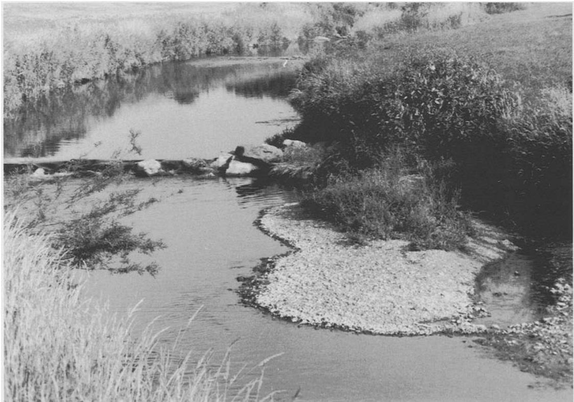
Fig. 11. Restructured Melk River: A gravel bank develops within a widened cross section downstream of a groyne and offers shallow water areas with smooth and inverse currents. The adjacent pioneer vegetation is restricted to the upper parts of the low flow channel; higher bushes and trees grow above the mean flow level.
