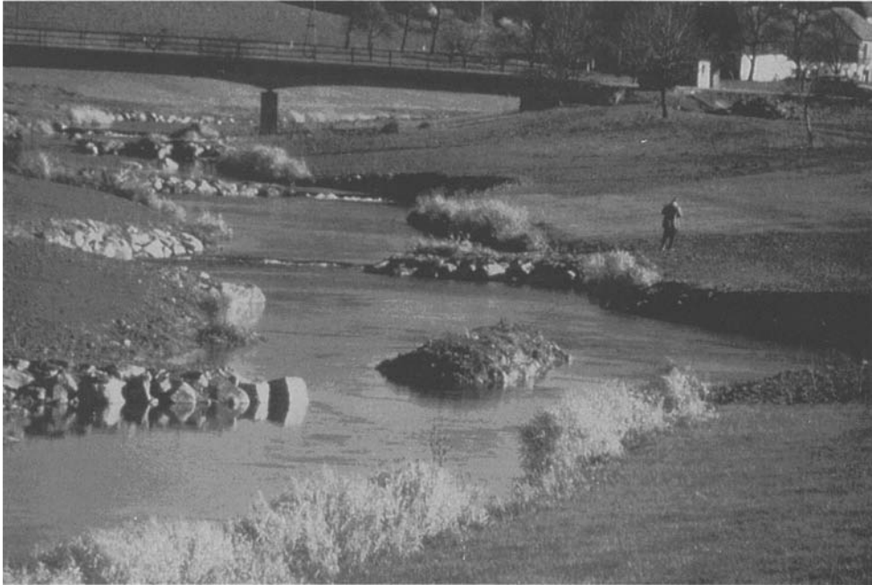
Fig. 2. After restructuring in autumn 1988 the Melk River shows a strongly increased spatial variety of the river bed (compare Fig. 3).
