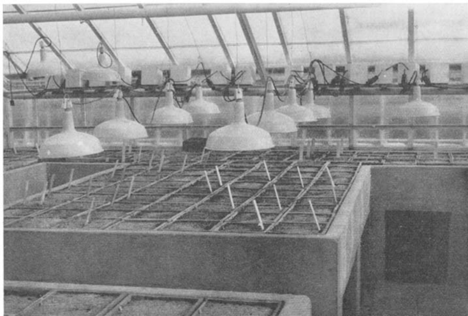
FIG. 1. AFTER EMERGENCE OF THE SEED EXTRA LIGHT IS GIVEN BY MEANS OF HIGH TENSION MERCURY LAMPS
