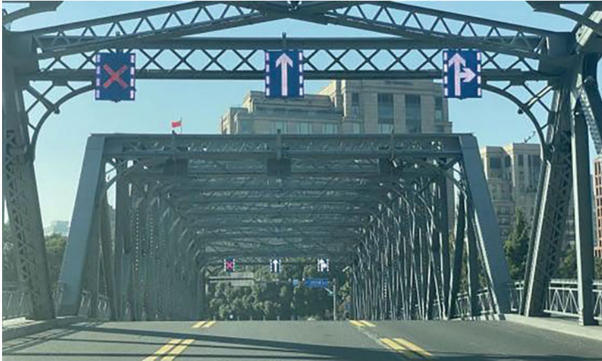
Fig. 5.3 Tidal lanes on the Garden Bridge in Shanghai with real-time guidance of driving direction using dynamic arrows
