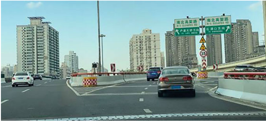
Fig. 5.1 Fork intersection approximately 25 m away from the ramp entrance of the Inner Ring Elevated Expressway and the North–South Elevated Expressway interchange in Shanghai, China
