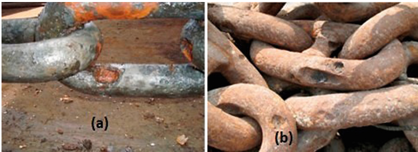
Fig. 4. Mooring chain with heavy corrosion cavities [1].
